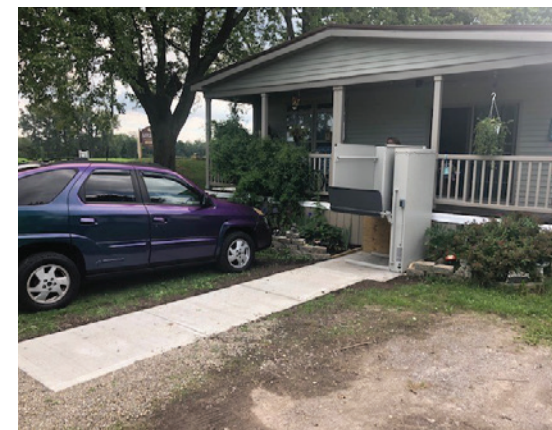
A recent exterior modification that was designed by Danise Levine.
