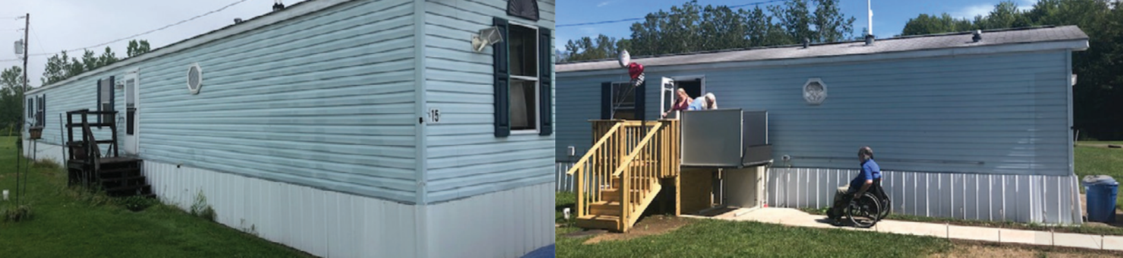
Gasport project: before
